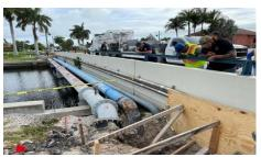
mains are supported by the concrete bridge piers and pipe hangers, the engineer will have to design the new pipe support. The three mains will be replaced as they are in very poor condition. The project kick-off meeting is scheduled for 9/10/21.
