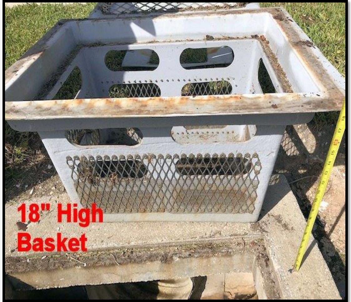
Filter Basket is Shorter Than Concrete Box
