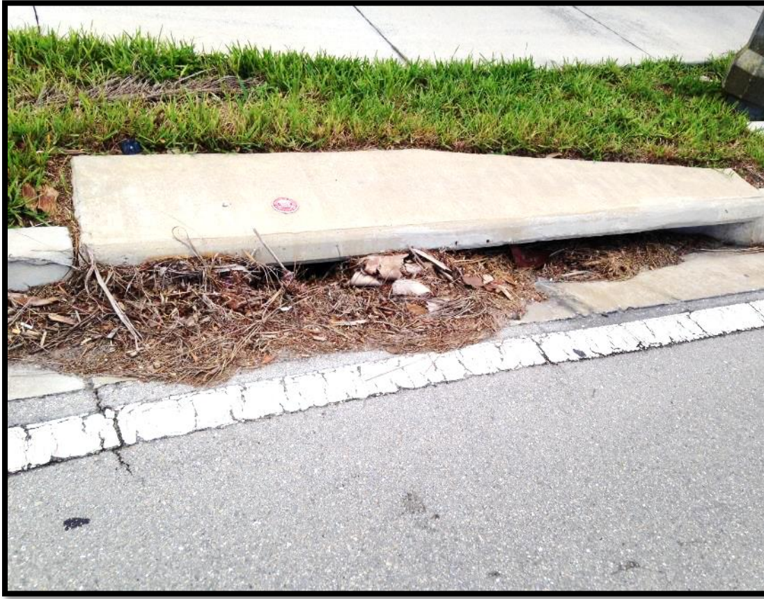
Organic material entering Collier Blvd Storm Water Inlet December 2018
