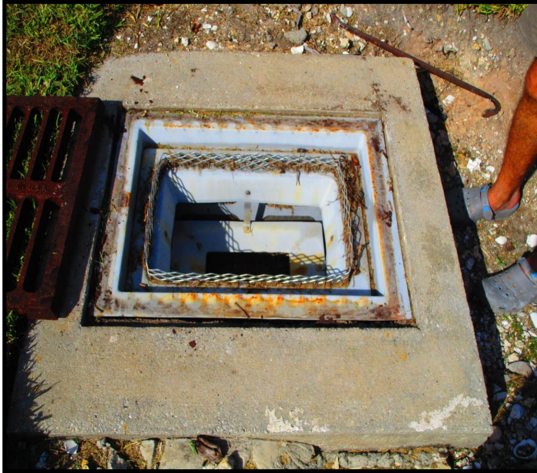
Filter Boom Missing
