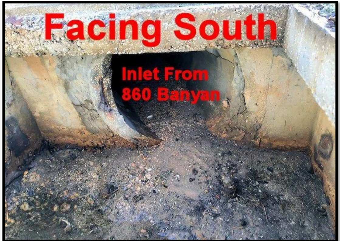
"Debris" is Sand & Gravel Blocking Pipe which accounts for most of the pounds removed as claimed by the City
