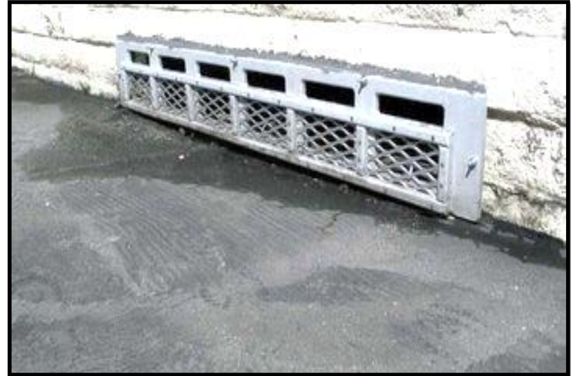
Install a suitable Grate barrier to eliminate large Organic debris from entry
