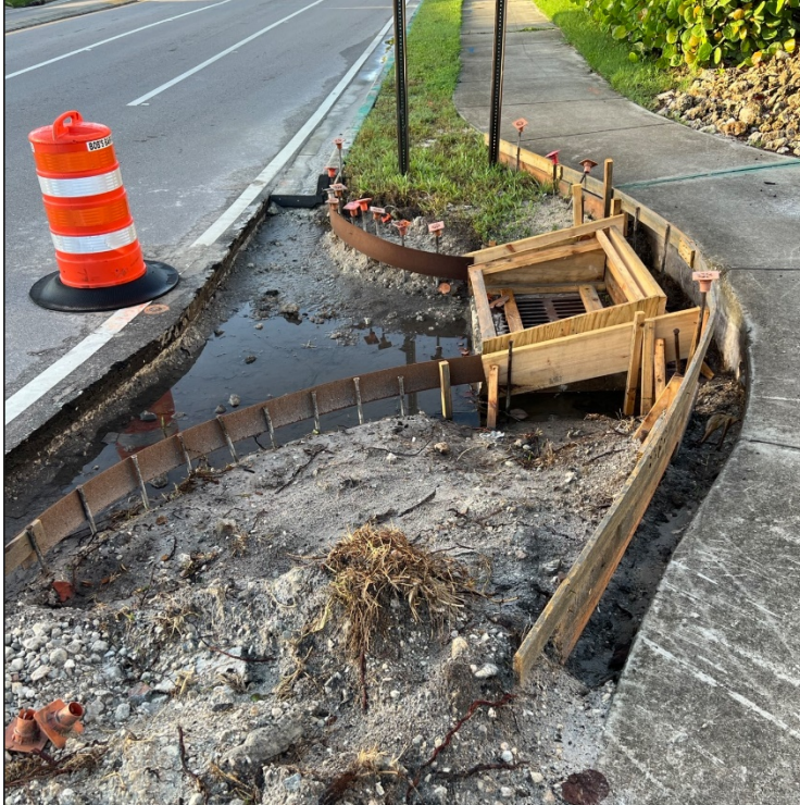
Forming of Cast-in-place drainage inlet on N. Barfield Dr.
