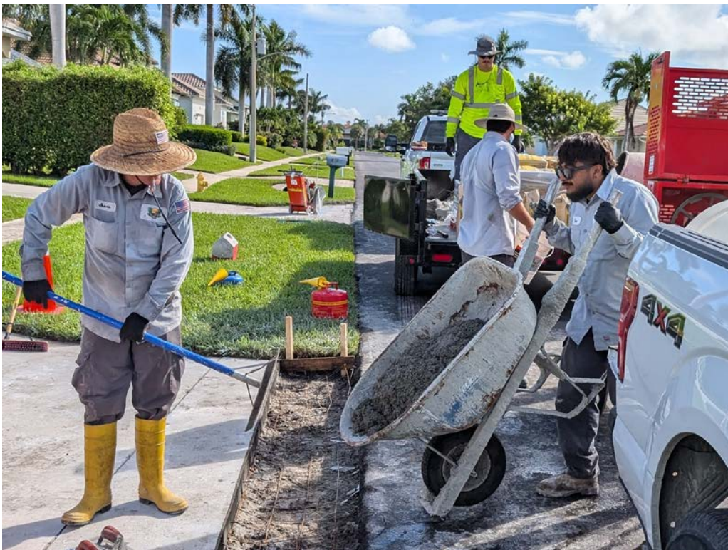
Public Works Crew constructing driveway elevation adjustment
