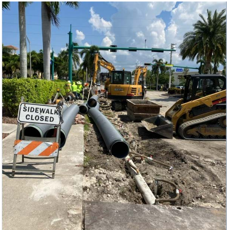
Drainage pipe installation on S. Barfield Dr.
