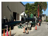
The contractor has completed replacement of the 20" raw water pipe with new HDPE piping. As part of the work, the contractor also upgraded the pipe cradles, connected the pre-filter using tapping saddles, and installed additional saddles for the chemical monitoring port.
