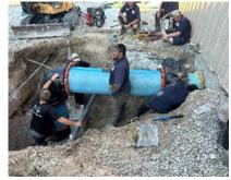
"soft dig," a method that reduces the risk of damaging surrounding infrastructure and utilities. Once exposed, the defective section of pipe was carefully removed and replaced with new material.
