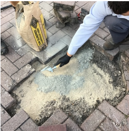
Brick Paver Repair on Collier Blvd near Marriott
