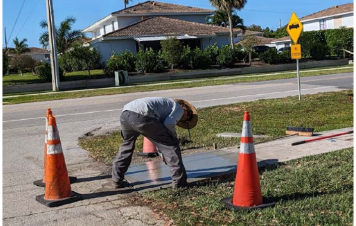
public works crew repairing sidewalk section
