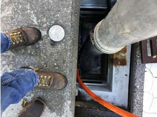
Yearly Storm Drain Filter Cleaning (MS4 Compliance)
