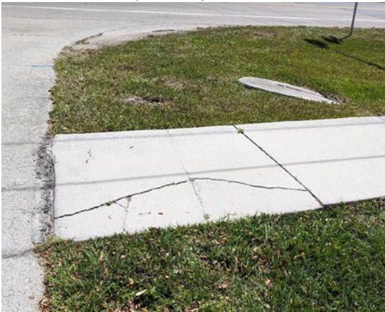
broken sidewalk repair at city annex
