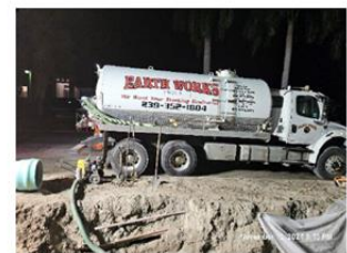
Left: Looking south on east side of N. Collier Blvd., Sewage is removed by pumper trucks (right picture) following the cutting of access holes in the FM.
