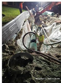
Left: Looking south on east side of N. Collier Blvd., Sewage is removed by pumper trucks (right picture) following the cutting of access holes in the FM.
