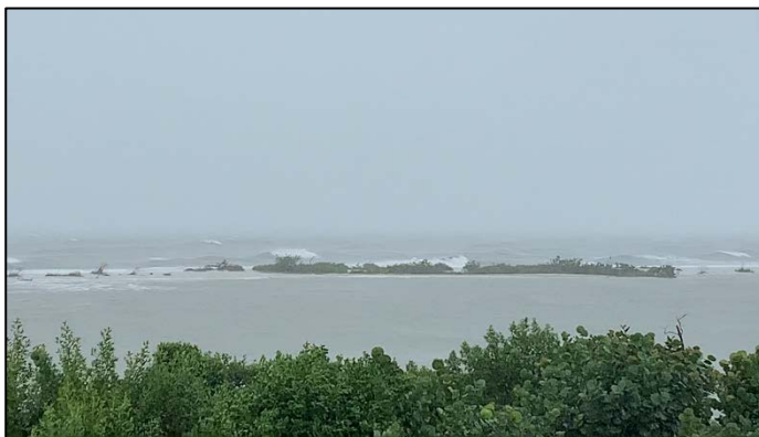
Figure 7: Sand Dollar Island berm dissipating wave energy from entering Tigertail Lagoon and Hideaway Beach
