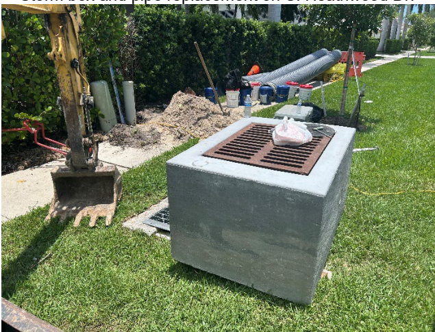
Storm box and pipe replacement on S. Heathwood Dr.
