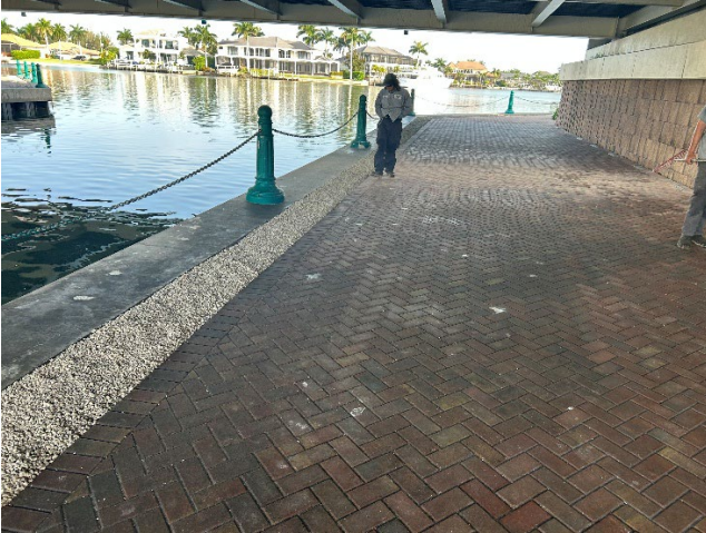
Herb Savage bridge stone replacement
