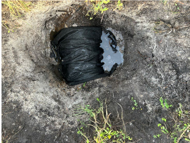
Marco Lake Dr. storm pipe repair.
