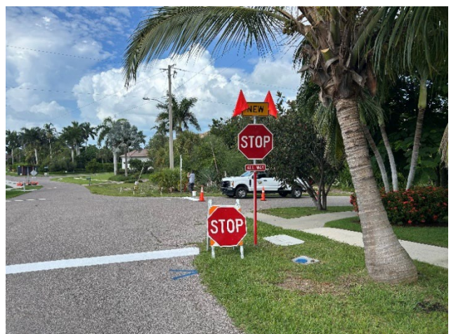
New stop signs installed at Inlet and Watson.
