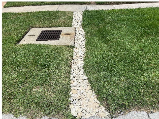
Leeward Ct. washout repair.
