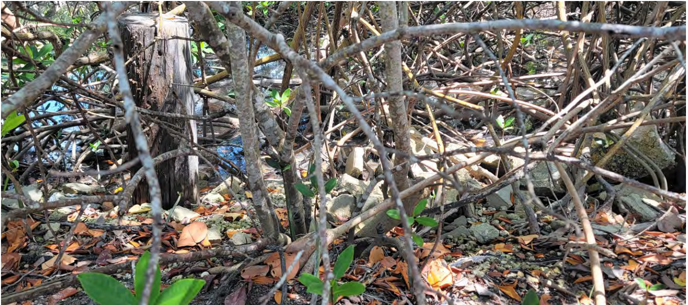
Figure 2: Riprap shoreline. Fill is landward of it and high tide is waterward.
