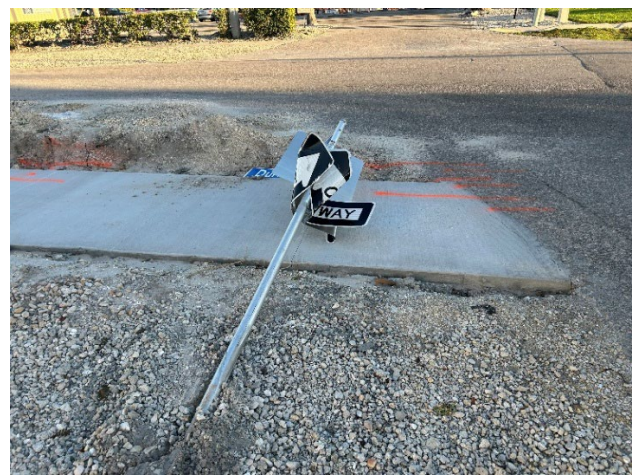
Dunford Lane sign replacement
