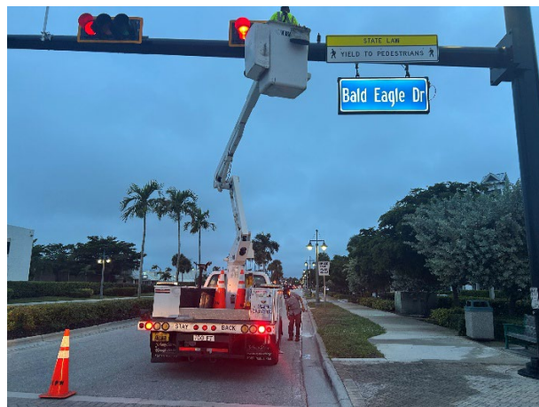
Traffic signal light replacement at Bald Eagle and Collier Blvd.
