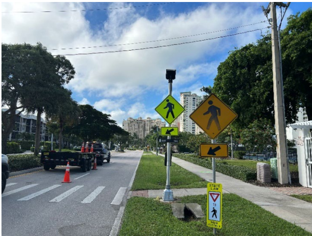
Crosswalk installation at Beach Club access
