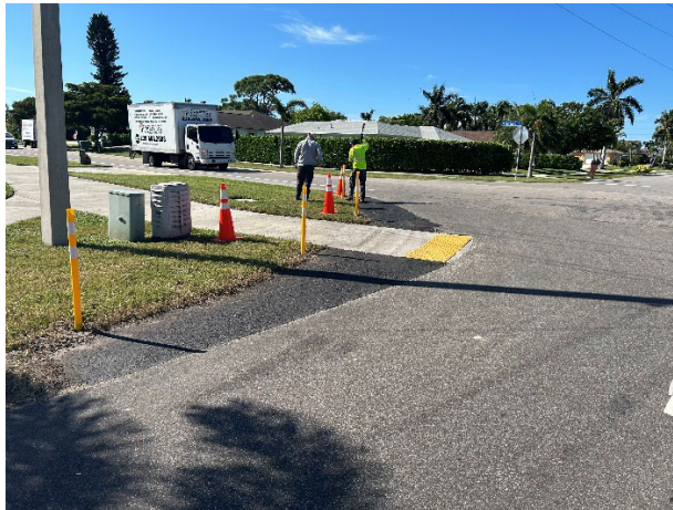
Edge of pavement repairs at Fairlawn and Waikiki
