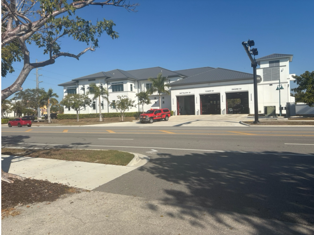
Figure 2: Marco Island Fire-Rescue Department (north)
