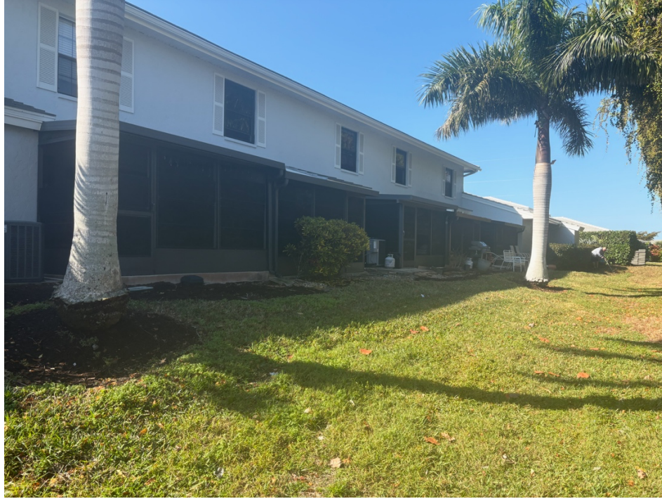
Figure 4: Backyard of 90 – 104 Marco Villa Drive residences facing the pickleball courts (south)
