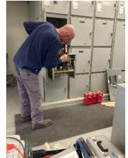
electrical system. Seeking expertise, we engaged a local electrical firm, which collaborated with Eaton Corporation, the breaker manufacturer. On April 18th, Eaton Corporation conducted on-site tests on the breaker, ruling out any issues with it and confirming the presence of a ground fault elsewhere in the electrical system.
