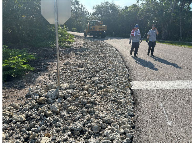
Reshaped ditch and installed riprap at Scott Dr. and Indian Hill
