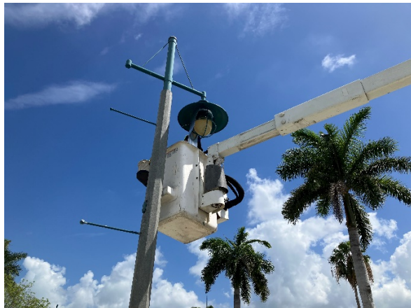
Storm damage repairs. Turtle shields and signage repaired.
