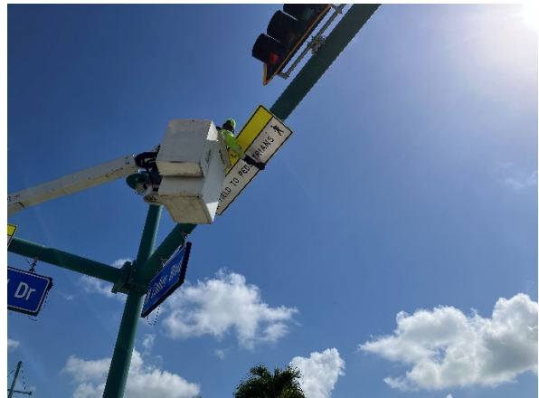
Storm damage repairs. Turtle shields and signage repaired.
