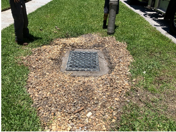
Stormwater outfall repair due to contractor cable damage.
