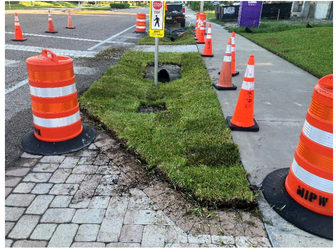
Installation of drainage pipe under shared pathway at 503 S. Barfield Dr.
