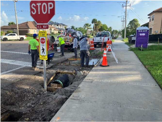
Installation of drainage pipe under shared pathway at 503 S. Barfield Dr.
