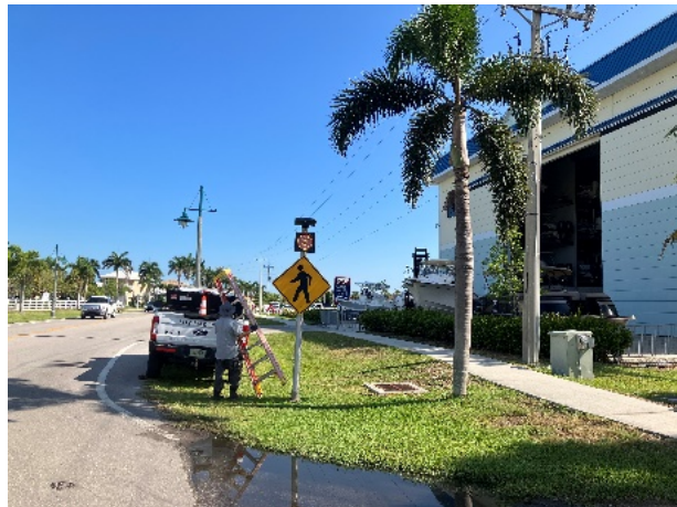
New solar flashing crosswalk beacon installed on Bald Eagle
