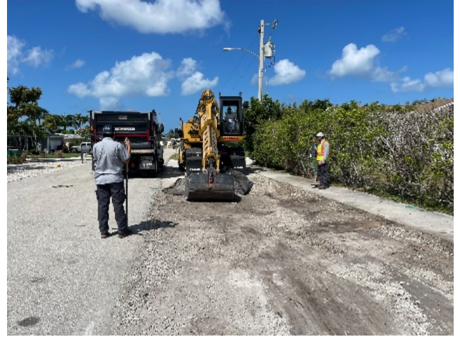
Before and after pictures of swale grading job at Bluebird Ave. & N. Barfield Dr.
