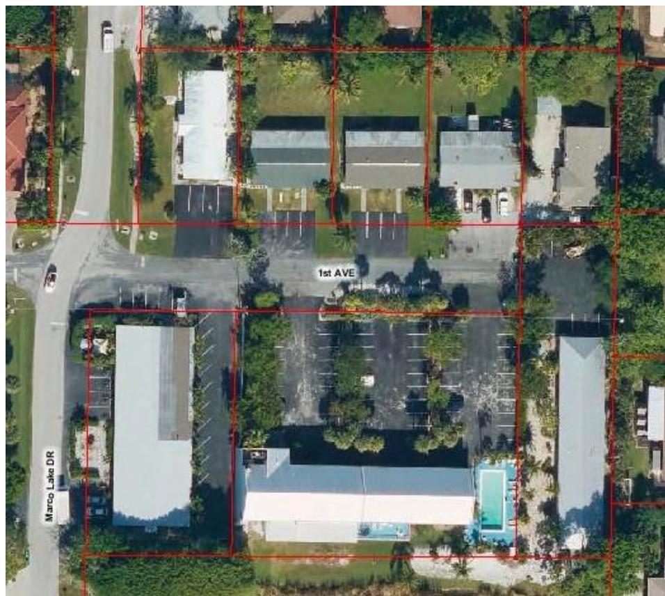
Figure 1 - Marco Lakeside Inn Aerial Image
