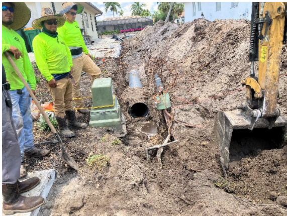
Repair of storm drain filter blockage issue on Cara Ct.
