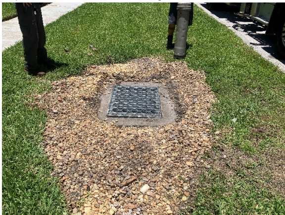
Repair of storm drain filter blockage issue on Cara Ct.
