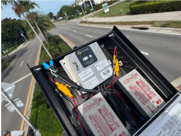
Flashing crosswalk electronic controler replacement on Collier Blvd.
