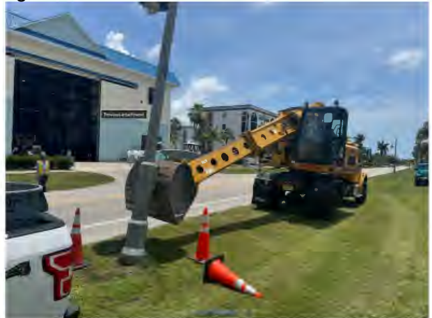
Light pole straightening at Rose Marina.
