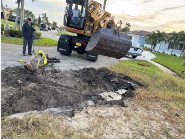
Old driveway pipe removed at Meadowlark Ct.
