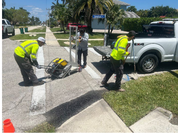
Edge of Pavement repair on Barbados and Gerranium
