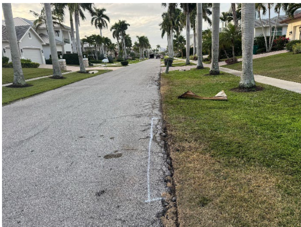
Edge of pavement repair at Hyacinth Ct.
