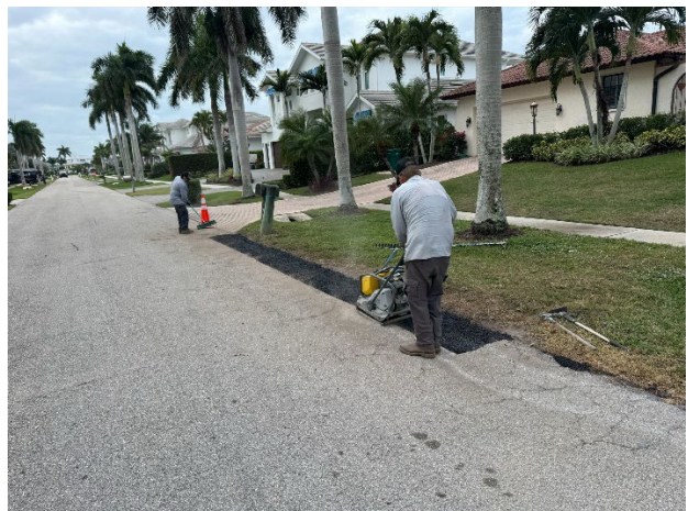
Edge of pavement repair at Hyacinth Ct.
