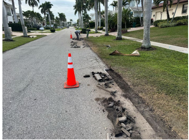
Edge of pavement repair at Hyacinth
