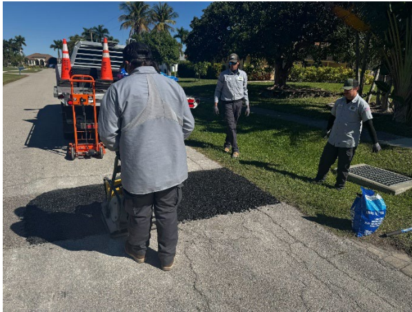
Bimini Ave. sunken road repair
