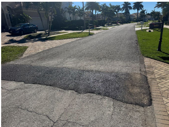
Bimini Ave. sunken road repair
