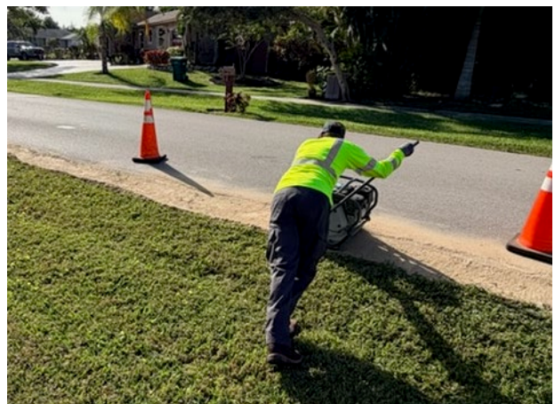
Edge of pavement repair at Hyacinth Ct.
