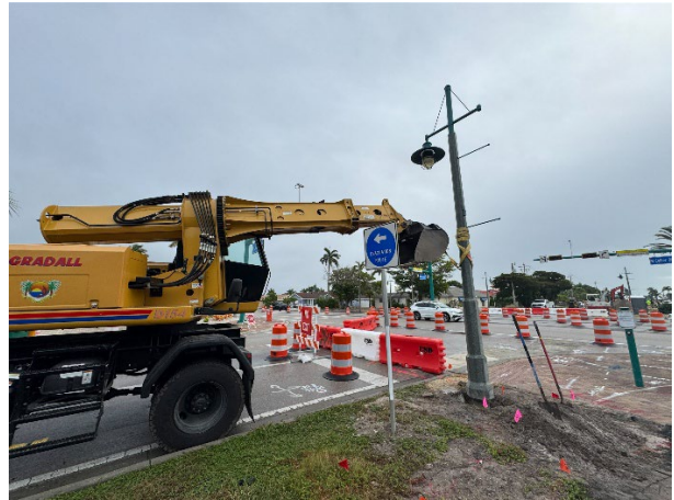
Light pole removal at Collier & Barfield
