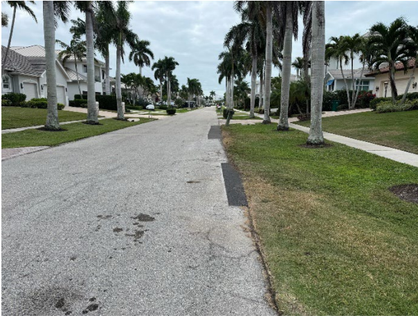
Edge of pavement repair at Hyacinth
