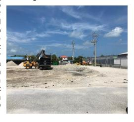
The contractor mobilized at the end of May and began with earthwork operations clearing gravel from the existing parking lot and excavating existing soils to prepare the site for construction. The contractor encountered and subsequently removed unexpected buried concrete pads, concrete blocks, and asphalt. Earthwork operations and building preparation is expected to be completed in the first week of July.
