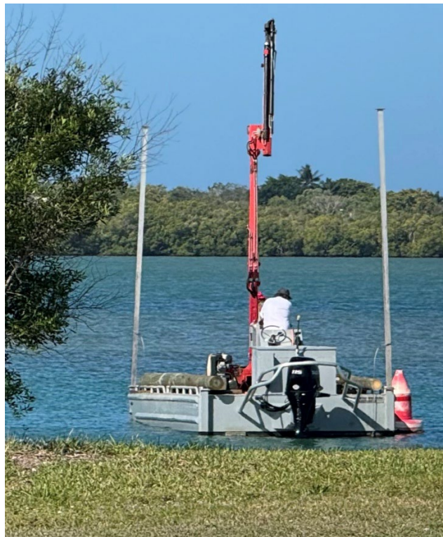
Waterway marker installation on Collier Bay
