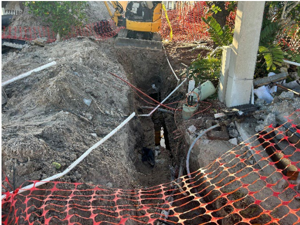
Storm pipe repair on Swan Ave. (relined storm pipe)
