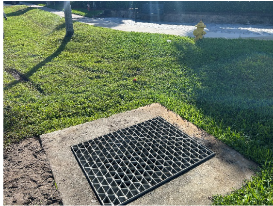
Storm box repair at Chalmer Bald Eagle
