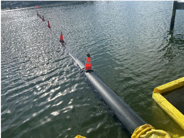
Storm pipe repair on Swan Ave. (relined storm pipe)
