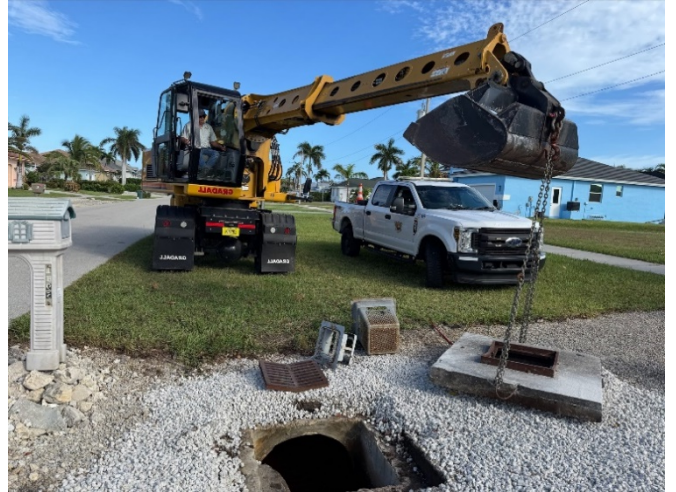
Leland Way Storm Inlet Repair
